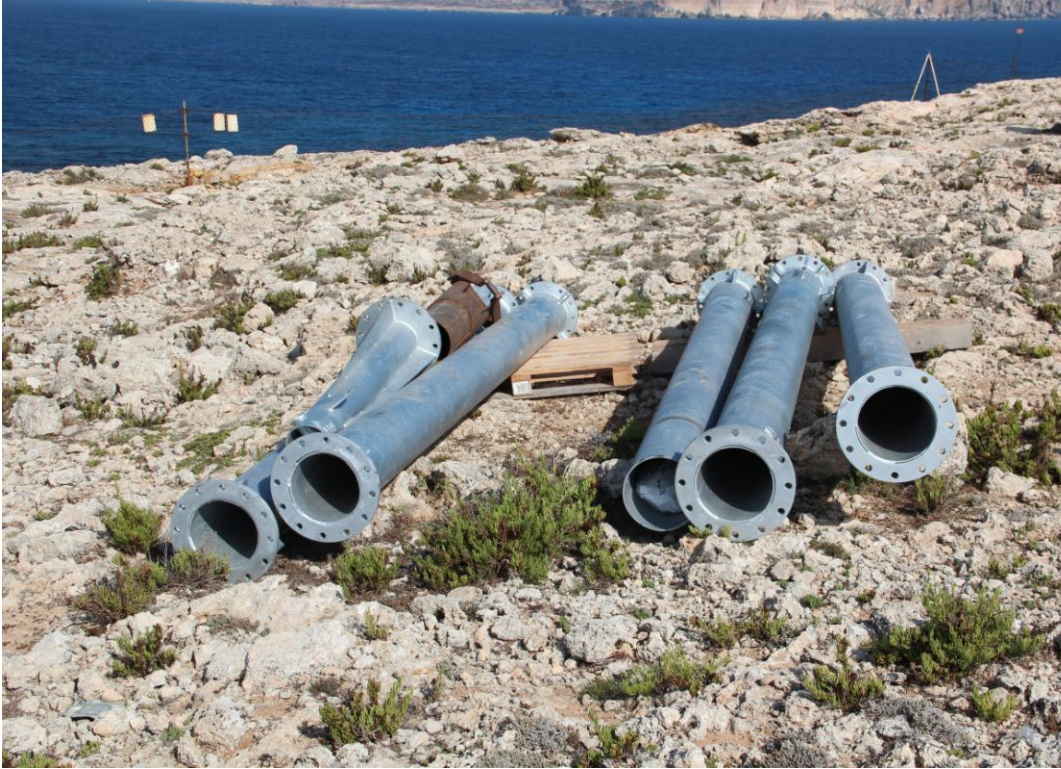
Figure 3 – The replacement galvanized gin-pole components (The head, rusty component at the rear, is not available)
