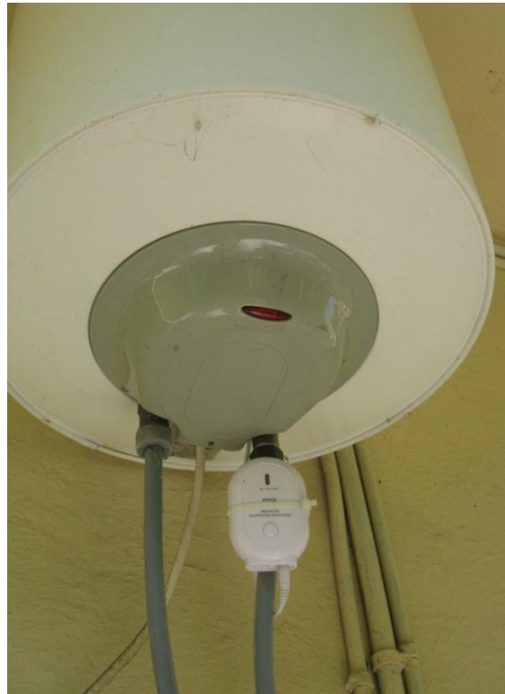
Examples of the equipment installation for the measurement of the electricity flow
