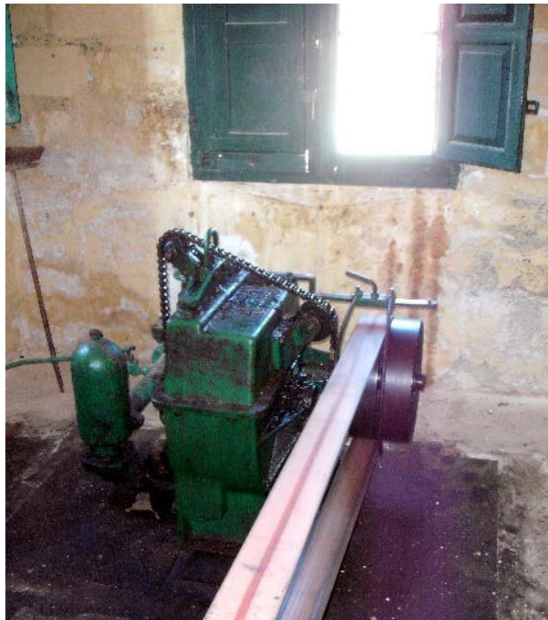
Figure 5. Water pump at the Comino borehole, having oily residues on the surface.
